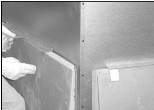
Figure 4.5 Unpacking Back Refractory
